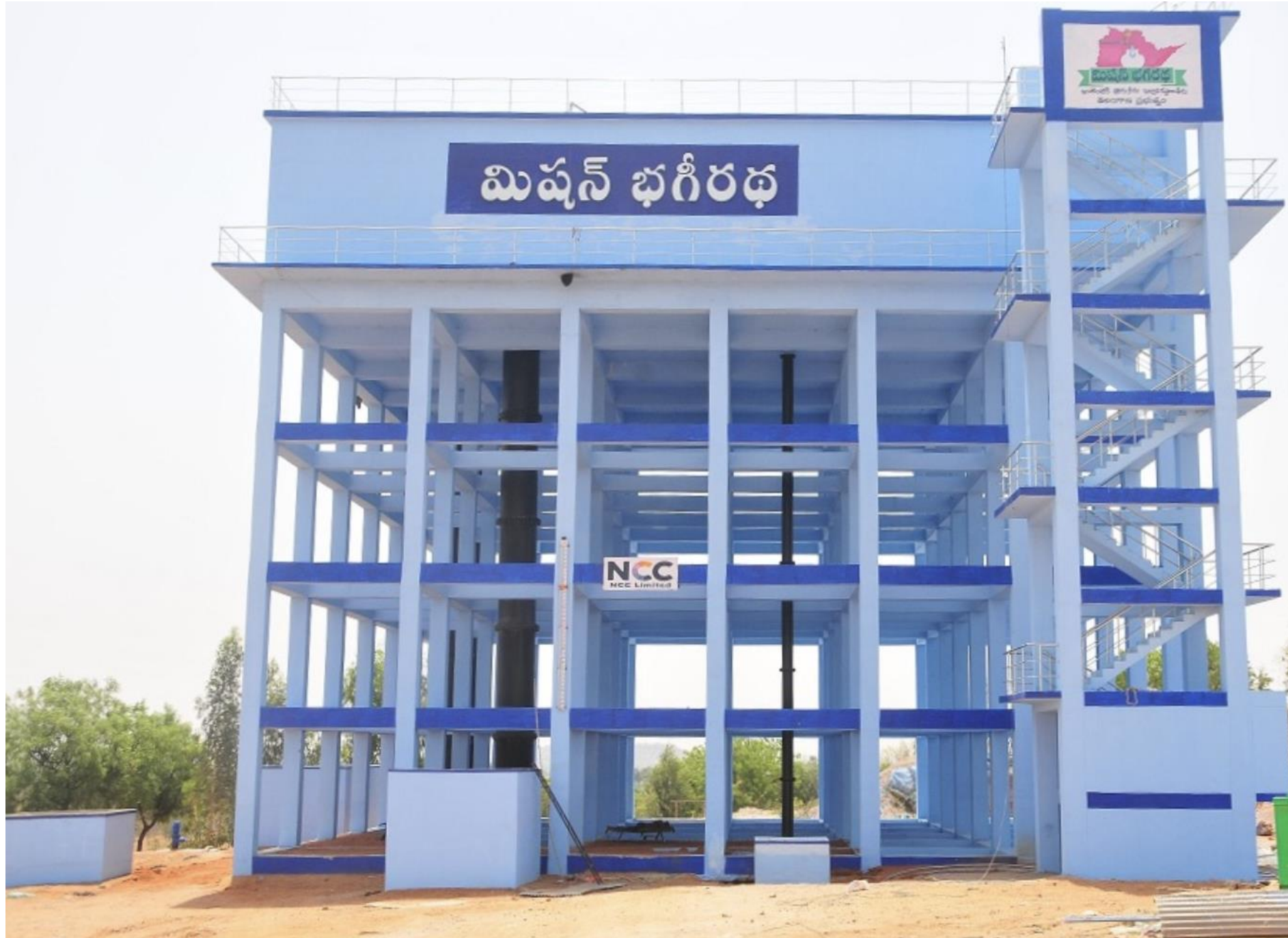
Over Head Balancing Reservoir
