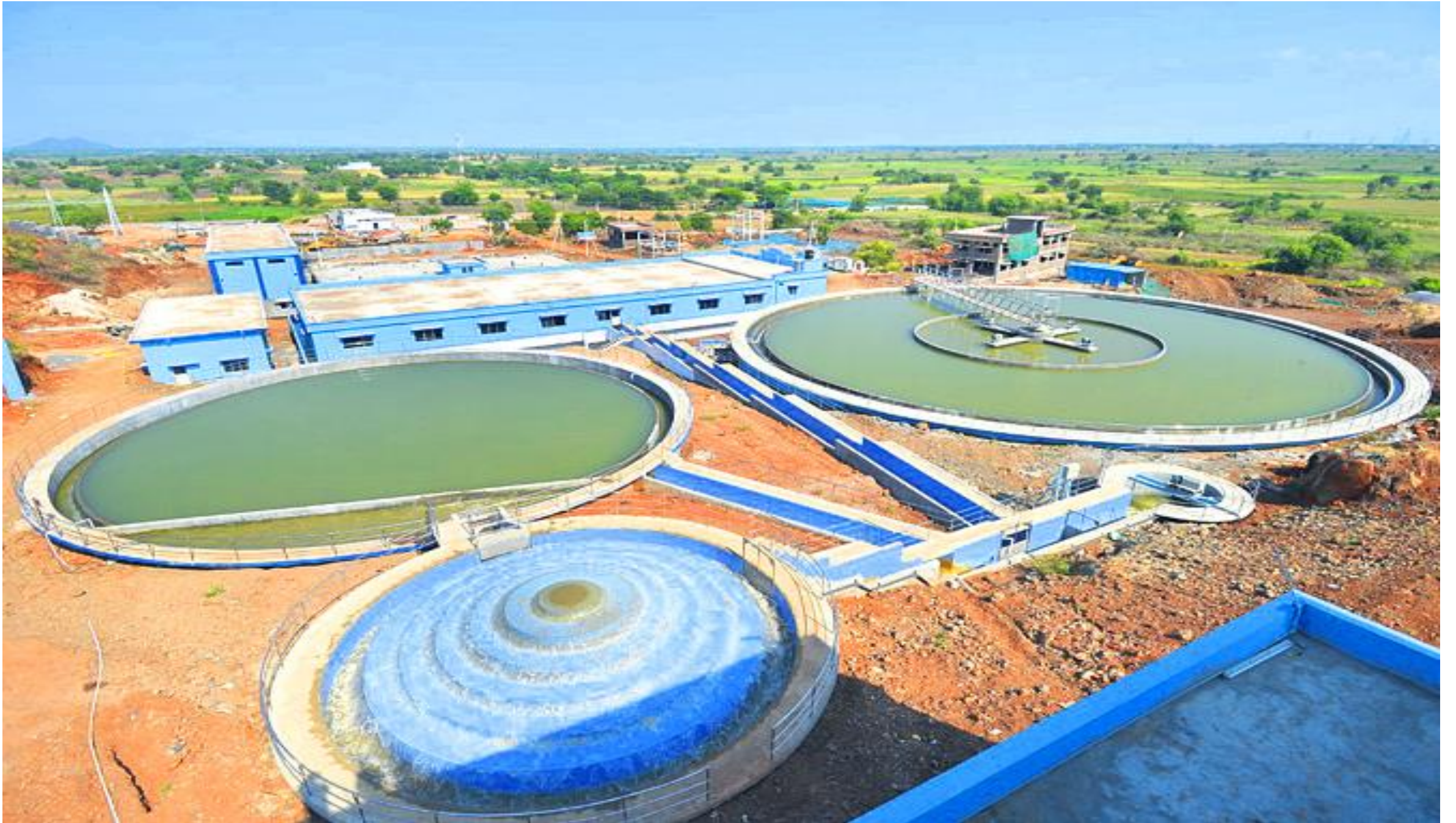
Water Treatment Plant constructed under Mission Bhagiratha
