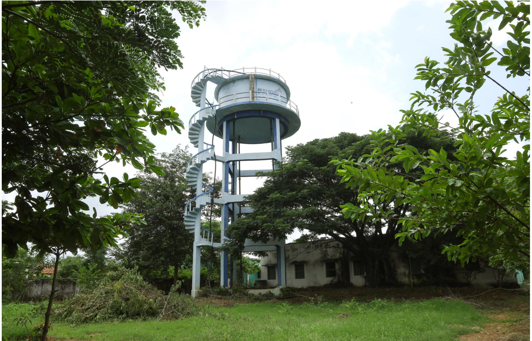
Over Hear Storage Reservoir in Village
